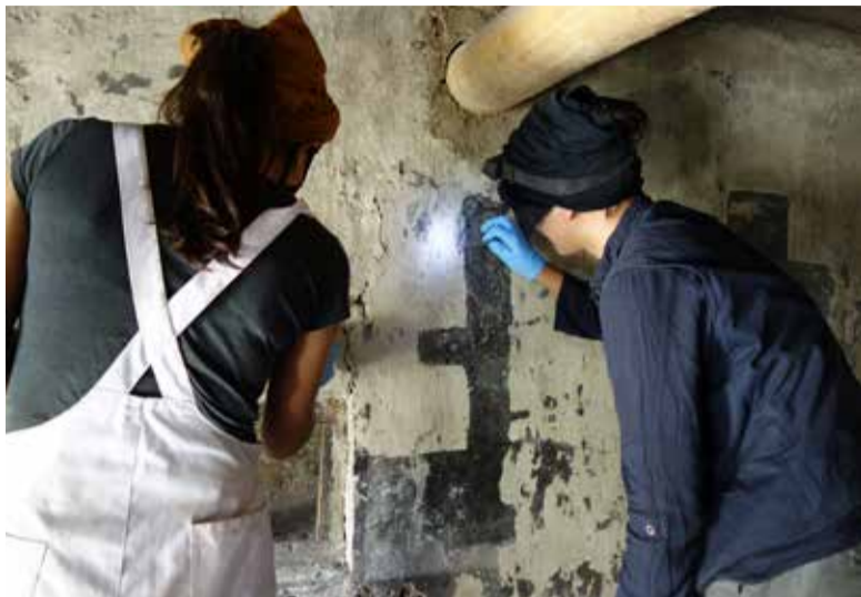
Conservator Noor Jahan and trainee Bhaga Tashi working at the LAMO centre, uncovering paintings under the white-wash (photo: Anne Voll).
